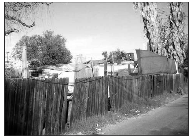
Trees not maintained, exterior fence in disrepair.
