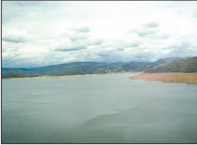
Oroville Dam, a So. Calif. water resource, is located on the Feather River in the north. Its lake elevation has dropped below the sensor level (704.09').
