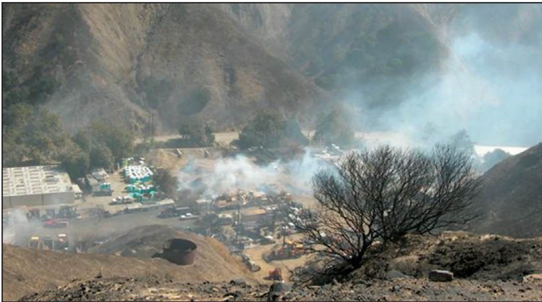
Commercial Buildings destroyed in Merek-Lopez Canyon fire
