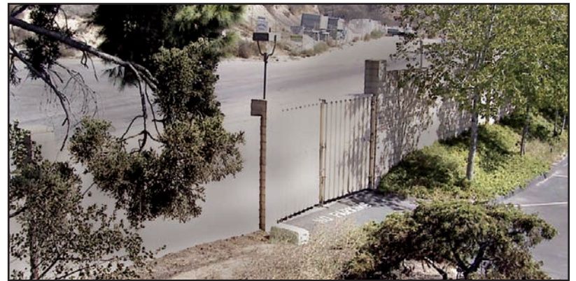
Blue Star Mobile Home Park Emergency Gate
