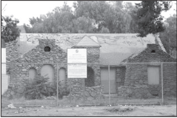
The Stone House, 8642 Sunland Boulevard prerenovation.
